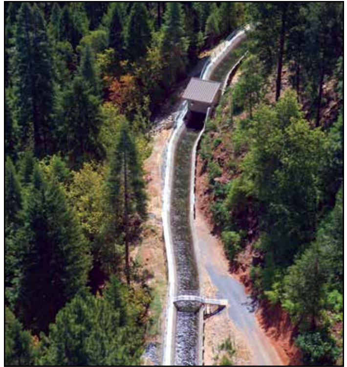
EID uses nearly 50 miles of canals, ditches, and flumes (pictured is a section of Flume 49/50) to convey water from high in the Sierra.
