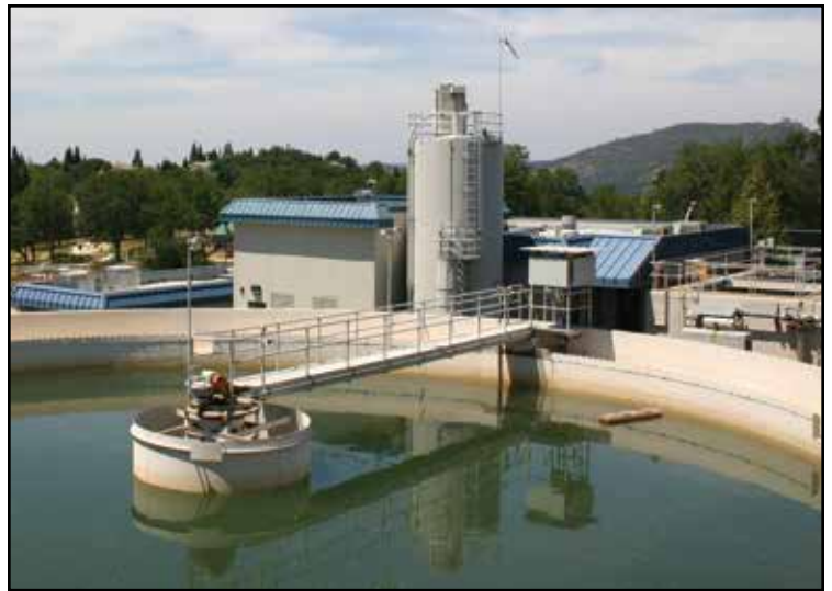
EID's El Dorado Hills water treatment plant is one of five treatment facilities in the district.
