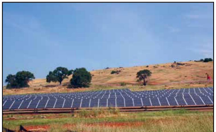
EID's El Dorado Hills wastewater treatment plant also includes a 1-megawatt solar facility that saves up to $250,000 a year on the district's electricity bills.
